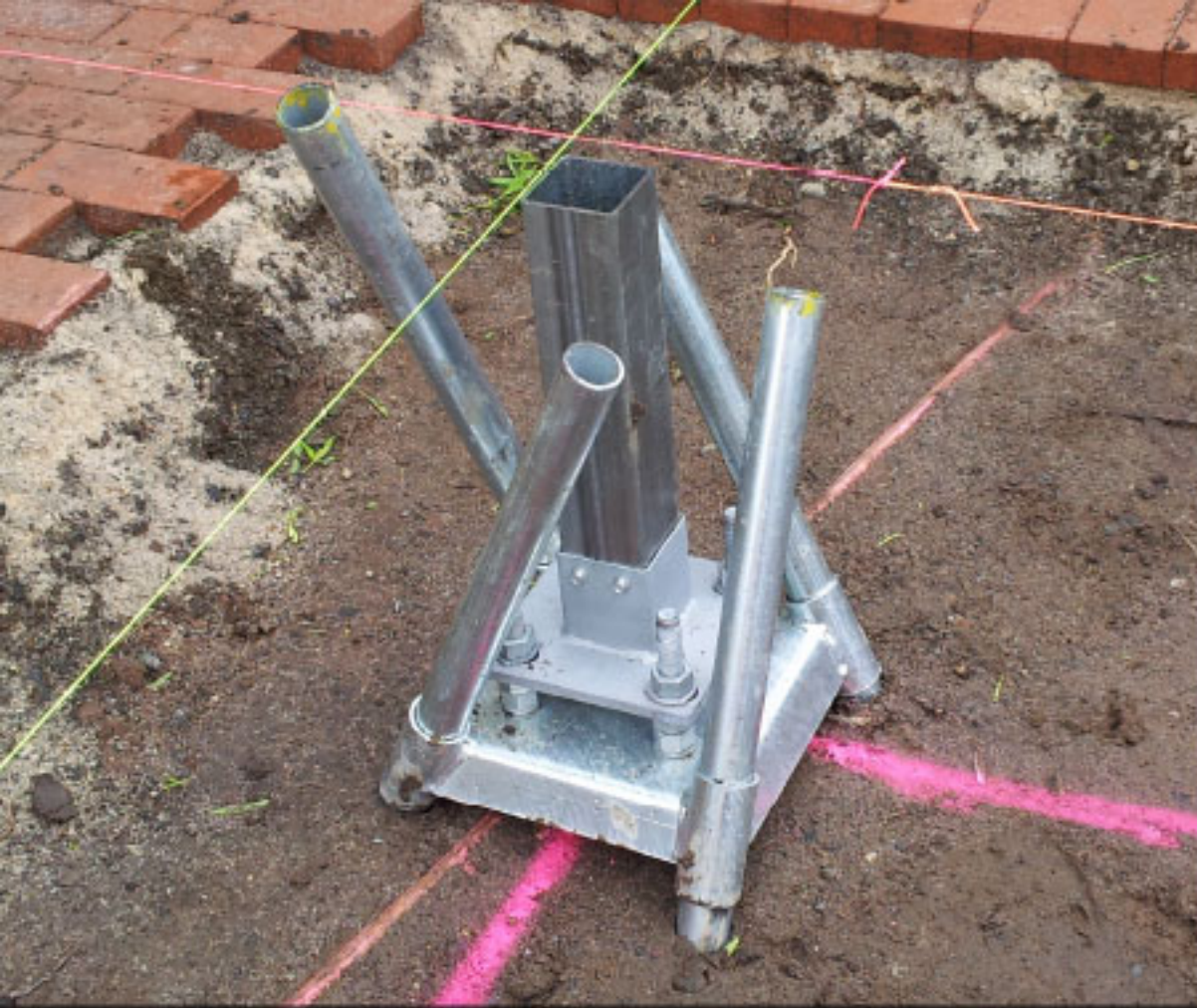
SF200 with fully adjustable stump assembly - Domestic Project
