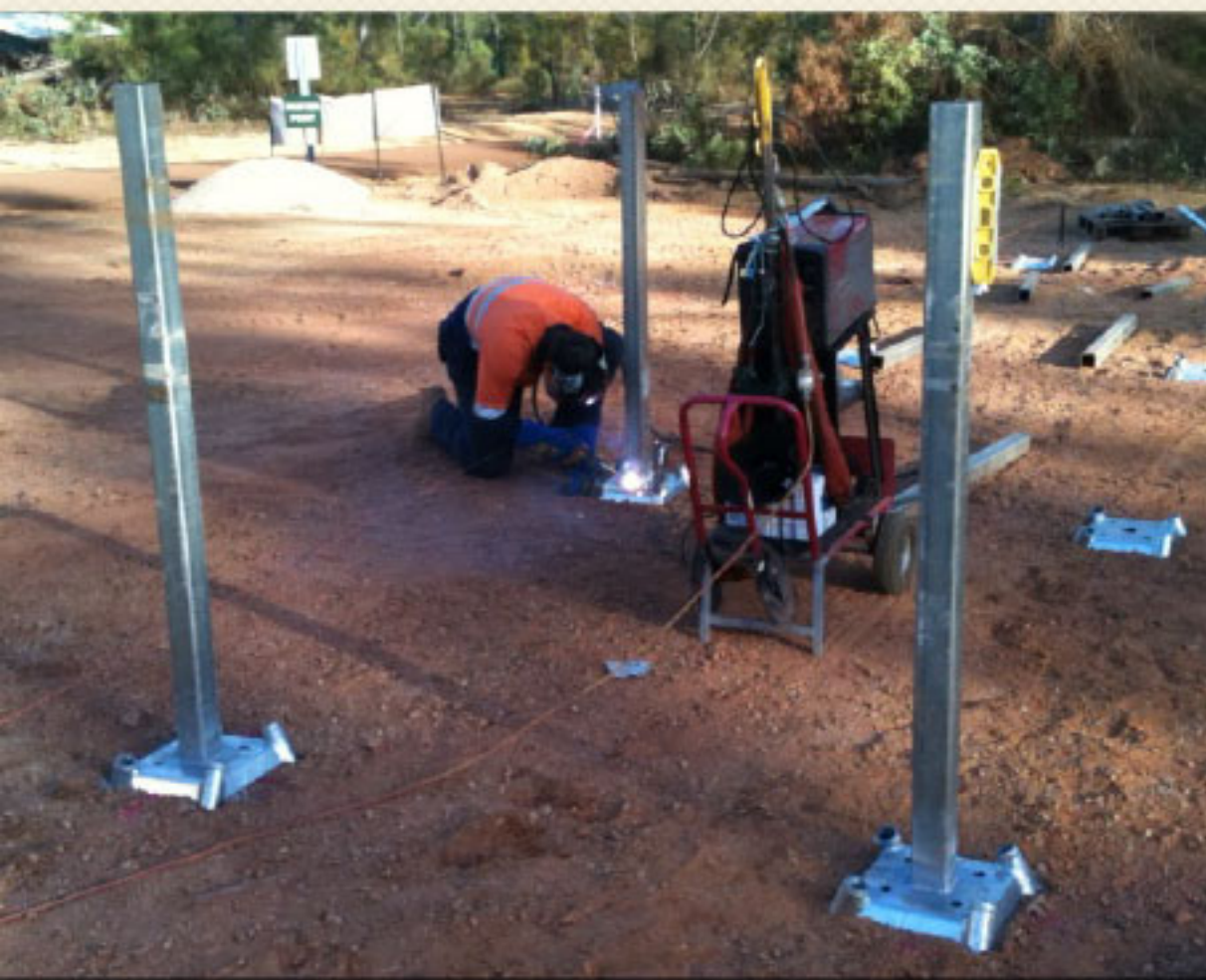
Welding directly to Surefoot
